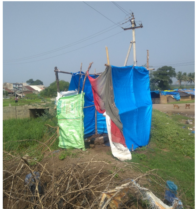
A temporary toilet in one of the residential areas
