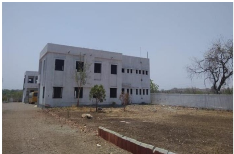
A school building being constructed at Shantivan
